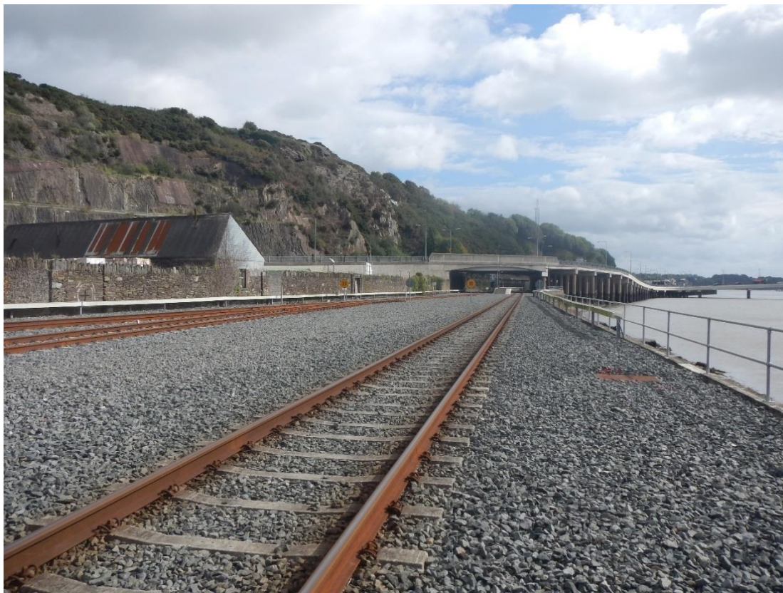
Plate 7.3 Buildings, railway tracks, roads, bridges, walls and other artificial surfaces make up a significant portion of the study area.
