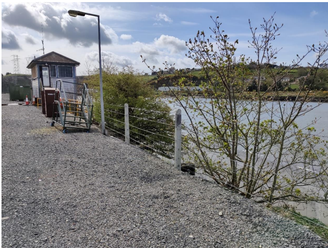
Plate 7.12 Signal cabin (left) at Ch. 1155 with connection to the River Suir.
