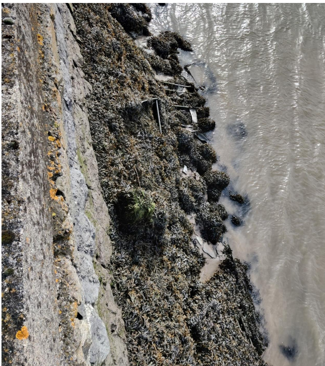
Plate 7.7 Existing quay wall surface with Fucus spp. community.
