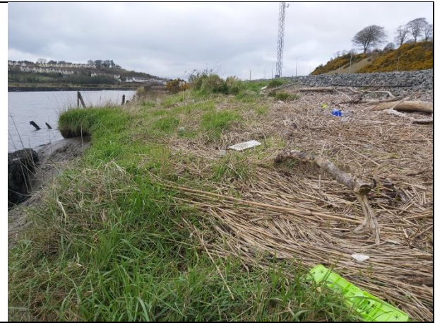
Plate 8. Grassland areas above retaining wall alongside railway
