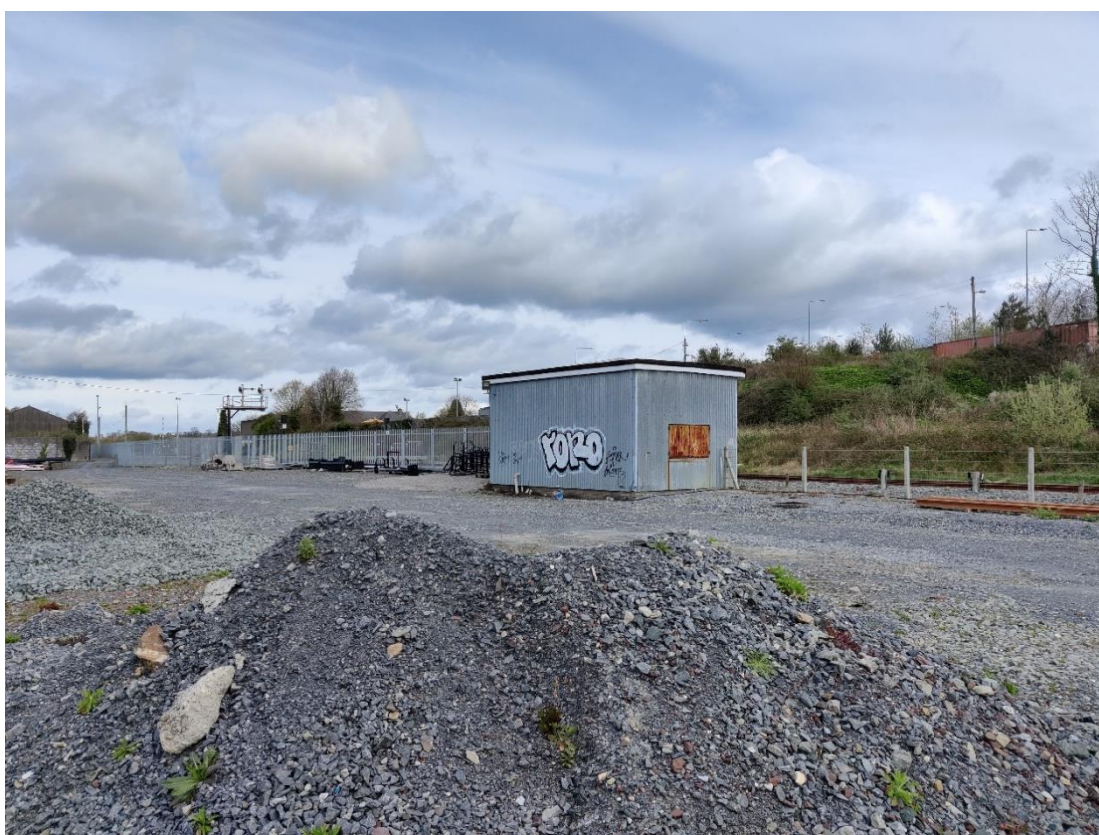
Plate 7.13 Disused building at the proposed location of the main construction compound.
